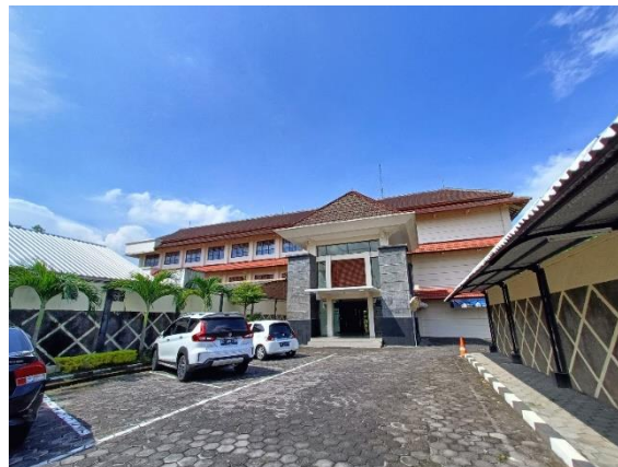
Figure 4. Campus Building 3 Section 1
