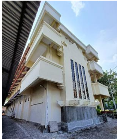
Figure 5. Campus Building 3 Section 2
