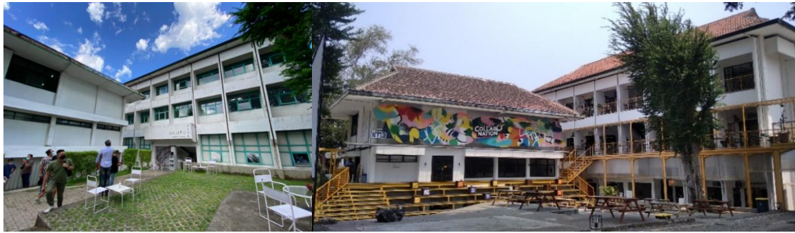
Figure 9 The Sculpture and Craft Building before Revitalization (left) and after Revitalization (right) (Source: https://archinesia.com/jnm-bloc/(2022) )
